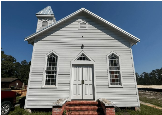
Reaves Chapel - Closer to Completion Every Day
